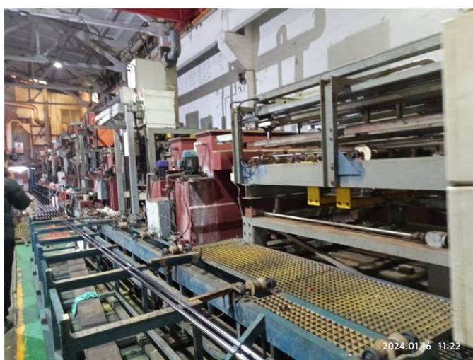
102 - External electroplating factory workshop
