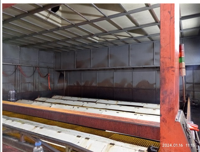
96 - External electroplating factory workshop
